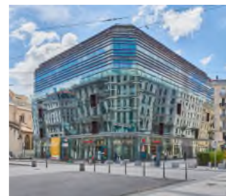
Lyon - Local commercial Place des cordeliers / © AEW
